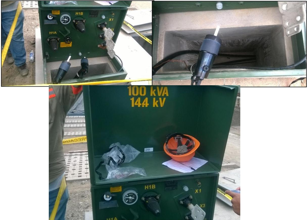
Figura 53: Pad-mouted monofásico de 100KVA.
