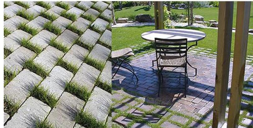
Figura 10: Adoquín permeable
