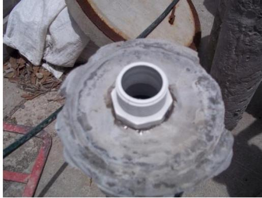
**Figura 8.4 Boquilla embebida de PVC**
