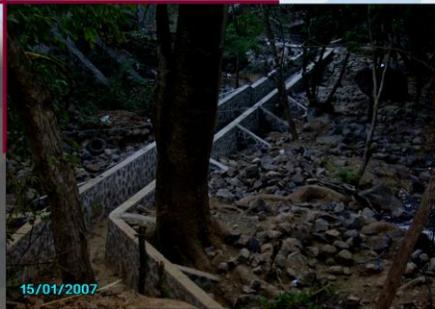
**FIGURA 3.9.1. CANALETA PARA EVITAR DESLIZAMIENTO EN LADERAS.**
