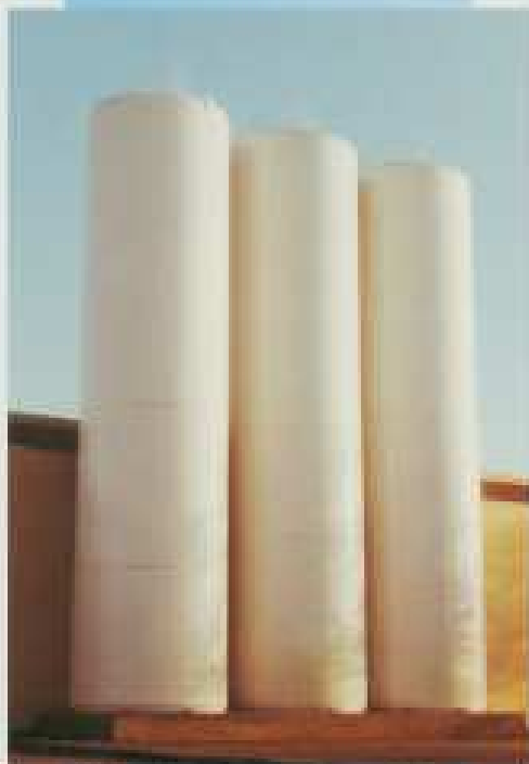
80,000 Gallon Silo Type Storage Tanks— custom painted exterior
