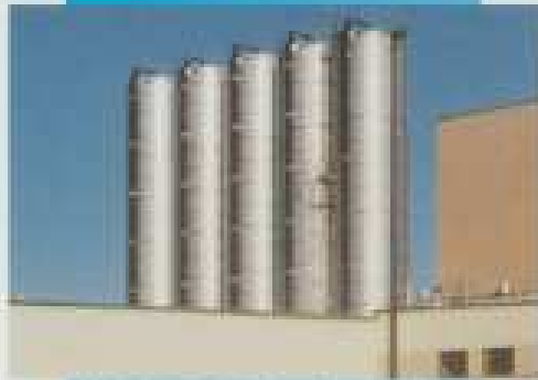
80,000 Gallon Silo Type Storage Tanks— stainless steel vapor jacket
