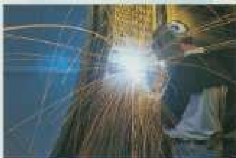
Experienced certified welders
