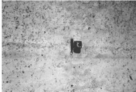
Fig. 2.7—Acceptable RCC pavement surface — Ft. Bliss, Texas
