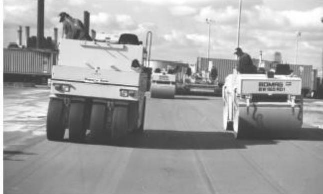
Fig. 2.3—Rubber-tired roller compaction
