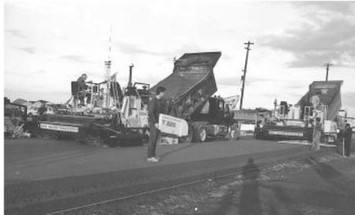
Fig. 2.1—RCC placement using modified asphalt pavers
