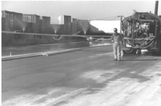
Fig. 2.4—Fog curing of freshly placed RCC pavement
