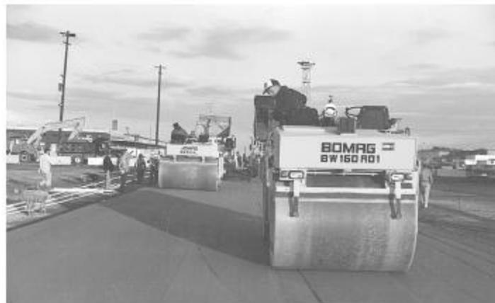
Fig. 2.2—Vibratory roller compaction
