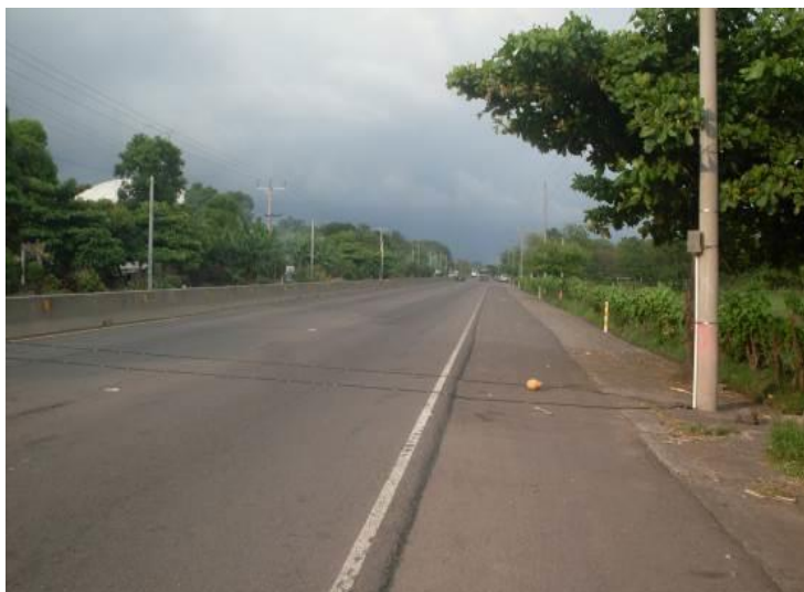
Figura 3.2: Pavimento Flexible Tramo I CA12S final del By Pass Sonsonate.
