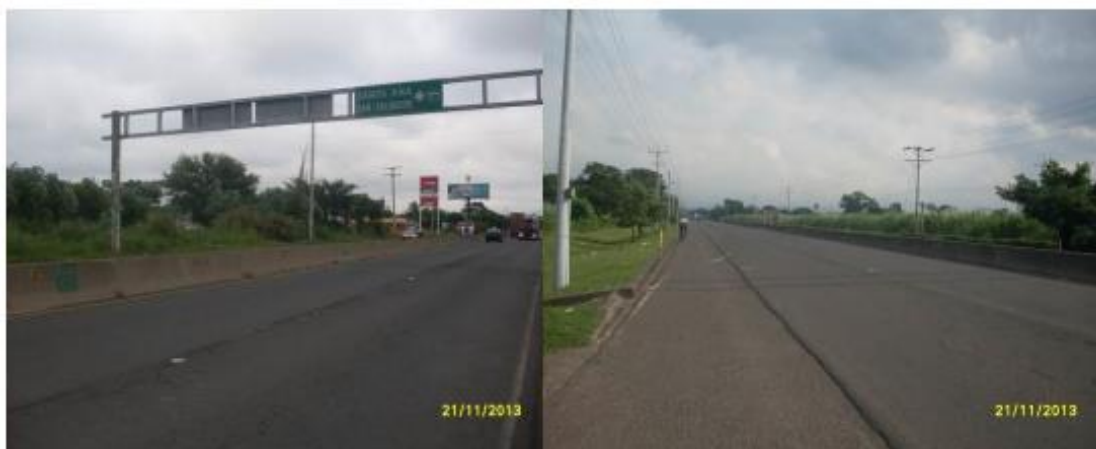
Figura 25 Pavimento Flexible CA12S final del By Pass Sonsonate.
