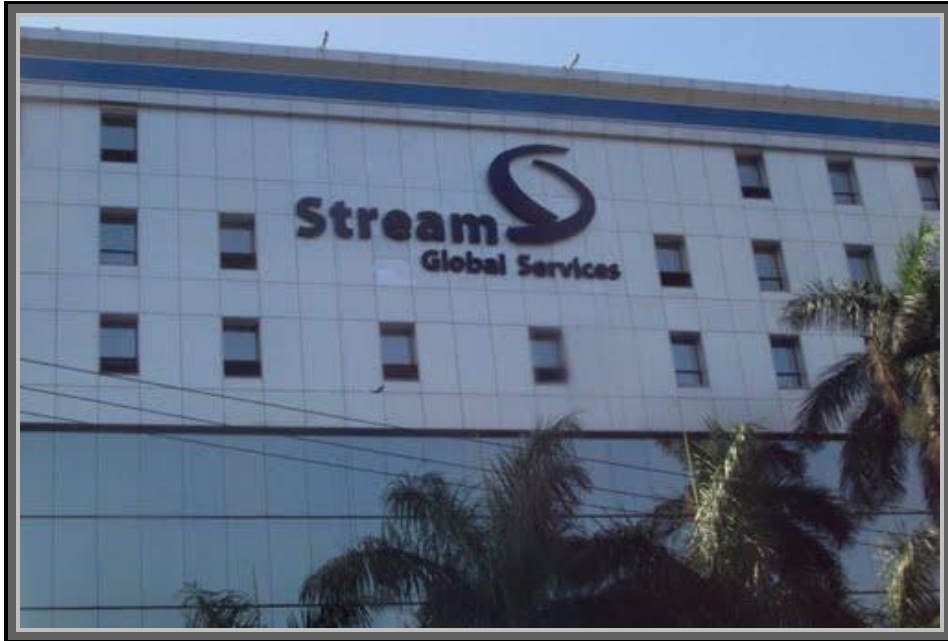
(7) Stream Global Services Building.
