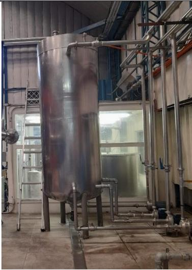
A large, vertical stainless steel tank is situated in an industrial facility. It is surrounded by various pipes, valves, and structural elements. The tank has a ladder attached to its side and is supported by a metal frame. | <p>Tanque de 500 galones que abastece las cabinas de producción 3, 4, 5 y 6 de la planta de producción INVIDA</p> |
