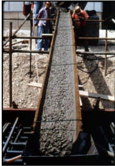
Figura tomada de: A Very Close Precursor of Self-Compacting Concrete (SCC).
