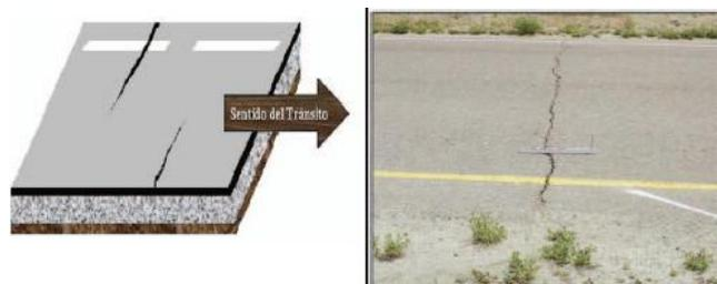
*Figura 3-8: Fisura Transversal*
